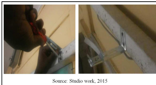
Figure 21. Fixing of frame holders.
