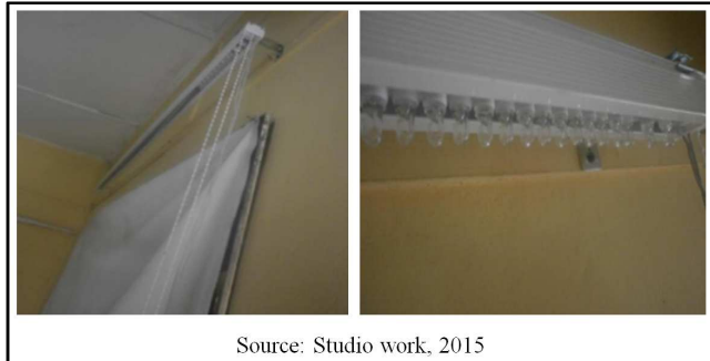
Figure 22. Blind frame fixed on holders.
